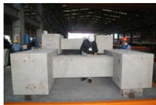
Construction of Specimen
